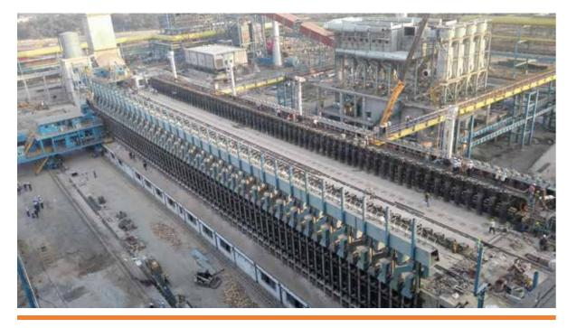
The JSPL coke oven plant, located in Angul, 160km northwest of the capital of Odisha State, will produce 1.9 million tons coke per annum. Sinosteel MECC's layout concept includes 4x72-chamber coke oven batteries, which is 4.3m TJL4350F type stamp-charging featuring twinfuel underjet, combination fired and waste gas recycling, 3-mtpa by-product facility, and 1.1-mtpa coke oven as well as coke quenching to be preserved.
